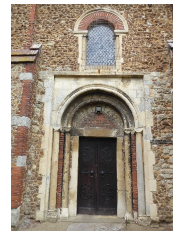
Figure 23 The south doorway of St John the Baptist church showing a variety of materials and detailing
