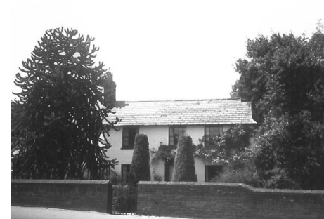
Figure 16 383 Old Road in 1985 (Essex County Council)
