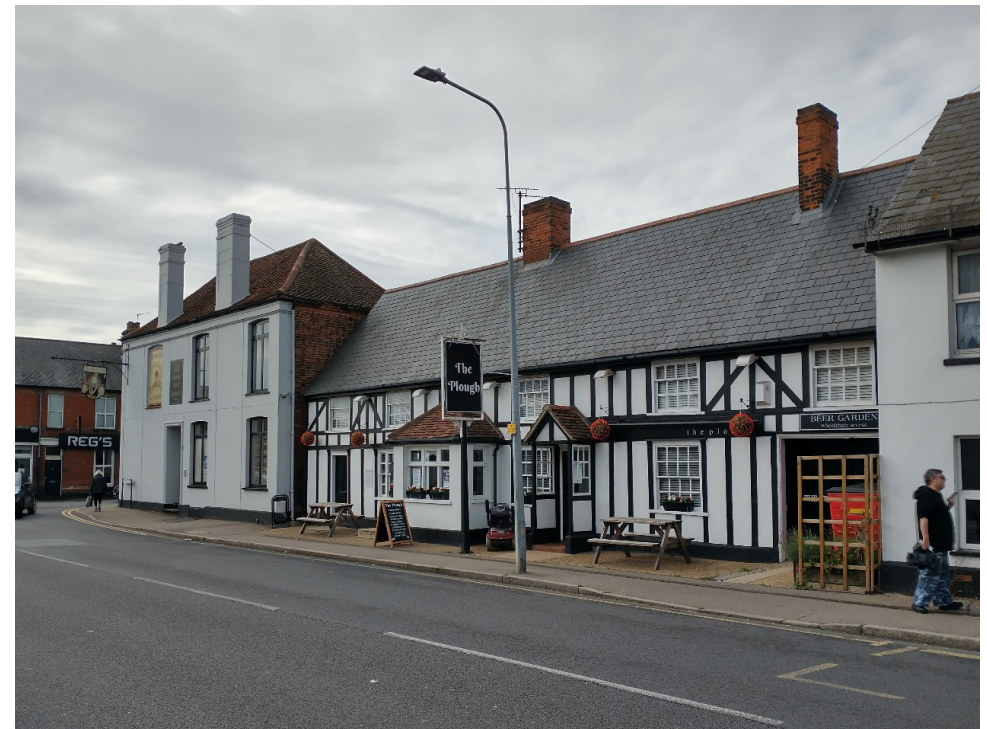
Figure 2 The Grade II listed Queen's Head former public house and The Plough on North Road
